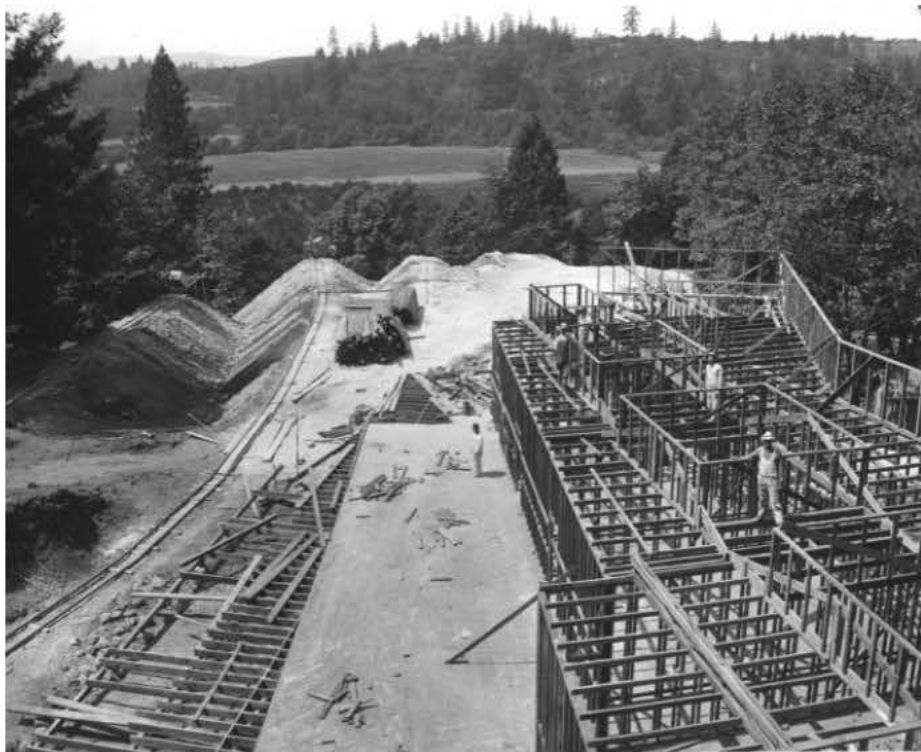
Construction of Irwin Hall (administration building), 1913.
